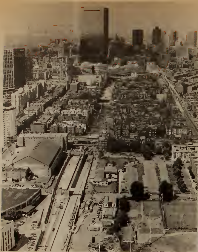
The Corridor looking north from the Massachusetts Avenue Station area.
